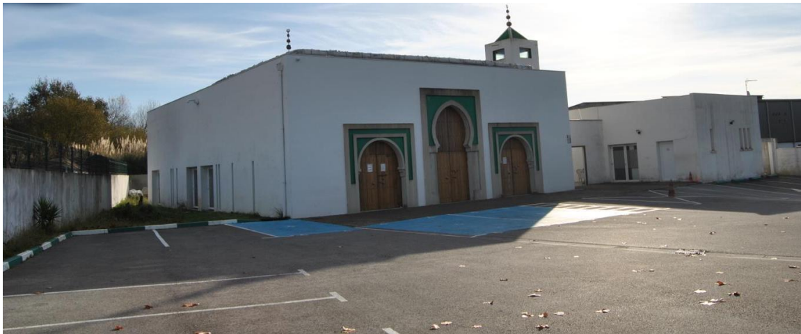
Figure 44 – View of the Bayonne mosque from the entrance
