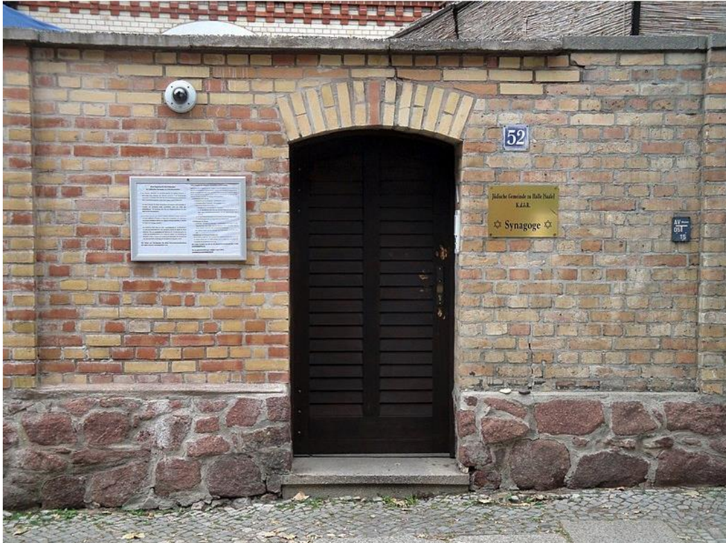
Figure 34 – Halle Synagogue’s side entrance
